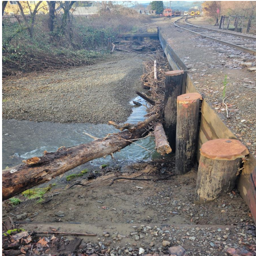
Broadbudd Creek Bridge, Willits: Before & After
