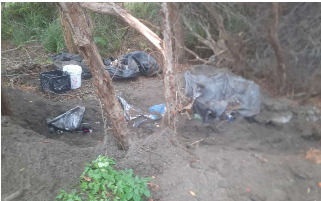
During: Below ground dump excavation
