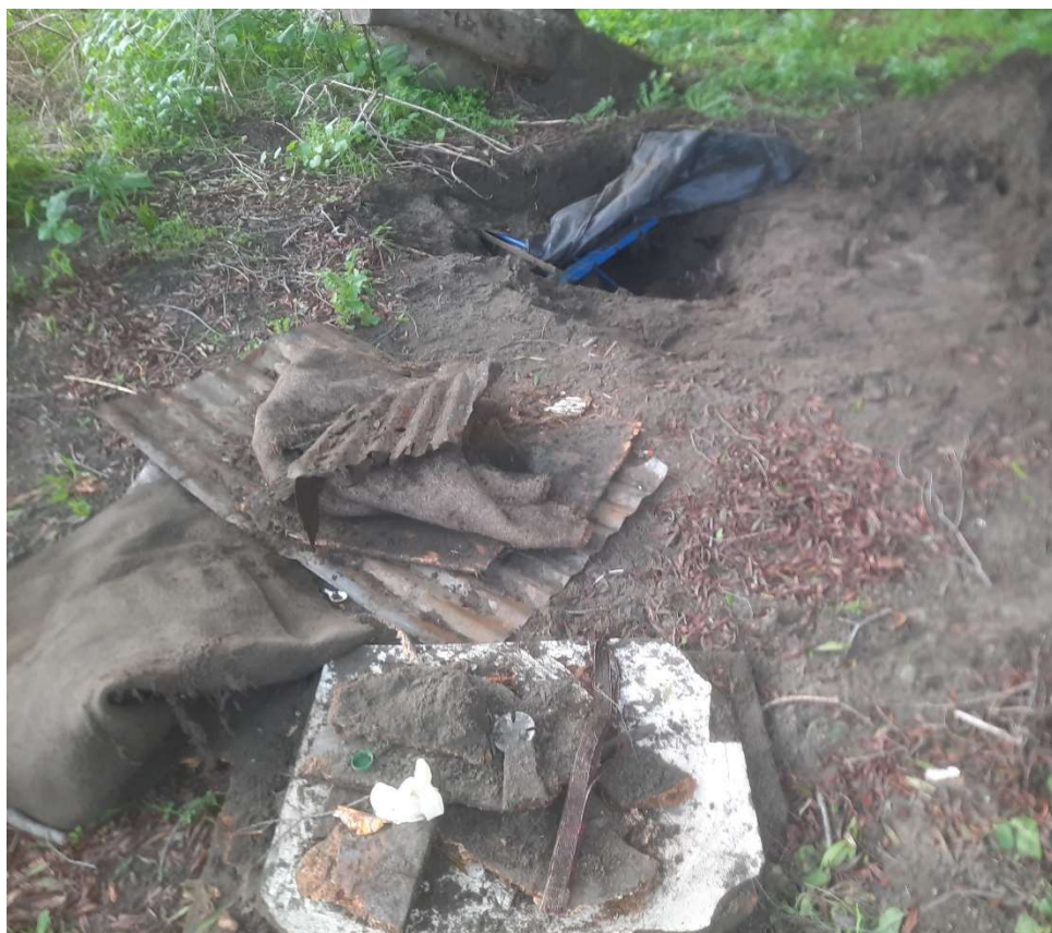
During: Below ground dump excavation
