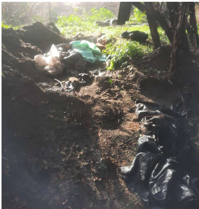
During: Below ground dump excavation
