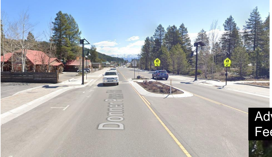
Roadway Reconfiguration Truckee, CA
